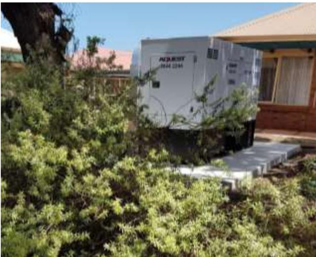
Although not programmed at this stage, the generator will be set up to automatically turn on at 10:00 am on the 1<sup>st</sup> of every month (running for 1 hour) and we will undertake a simulated power outage on an annual basis and run the generator for 3 hours.
